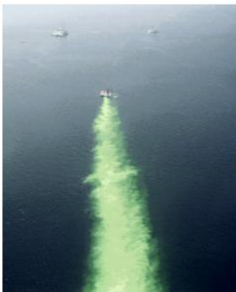
Example of spreading of dredged material in Øresund, Denmark
